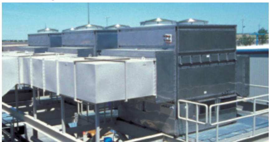
23. Performance of the ECOCool TIC system installed at a food processing plant in the California desert was significantly better than a conventional evap cooler with only a small increase in power consumption
